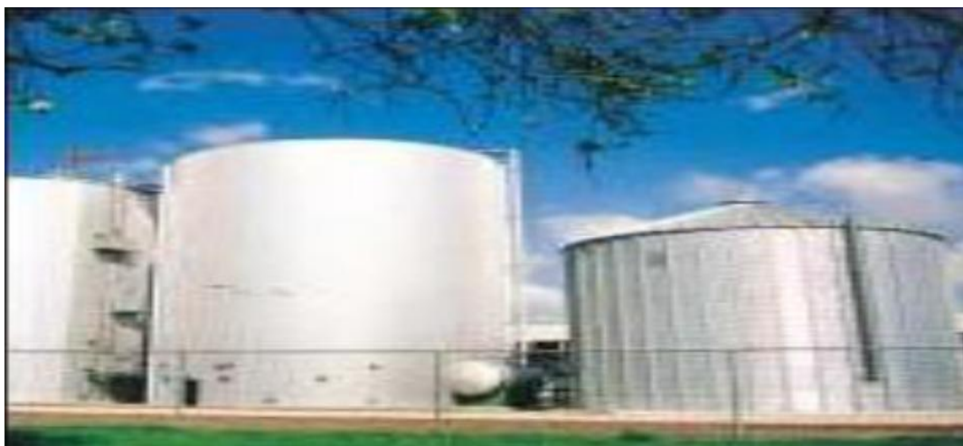
Figure 5: Anaerobic digester located at the Tilburg facility in the Netherlands.
