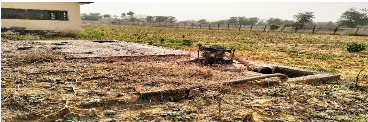
Plate 11: Soak away pit for slurry waste and water pump for spillage in the abature
